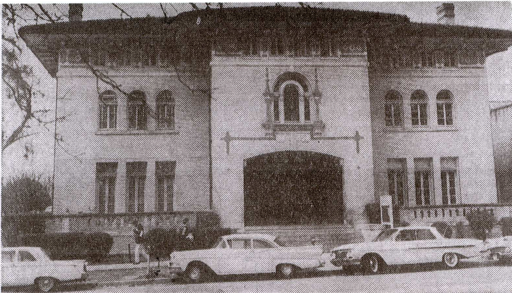
University of Texas YMCA-YWCA Building.
